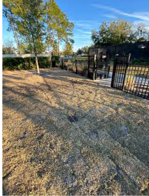
Sitework: Sod Repairs @ Maintenance Gate
