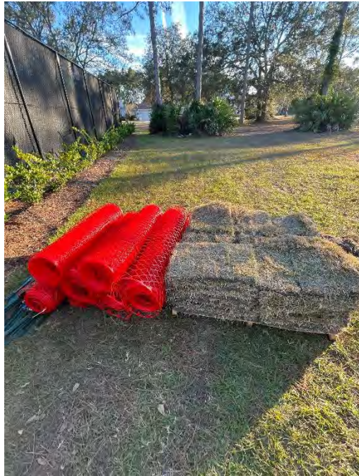
Sitework: Excess Sod & Temp Fence (pending)
