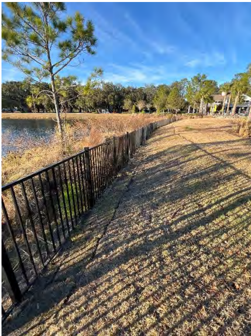
Sitework: Sod Repairs @ Fence Line
