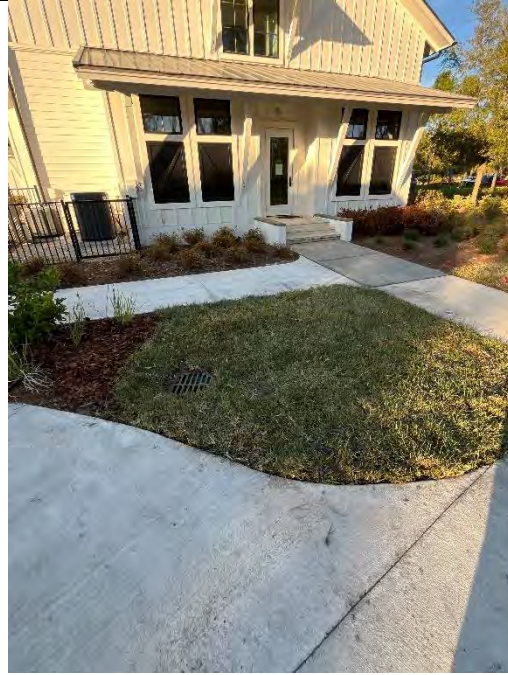
Sitework: Sod Replaced @ Gym Entry Door
