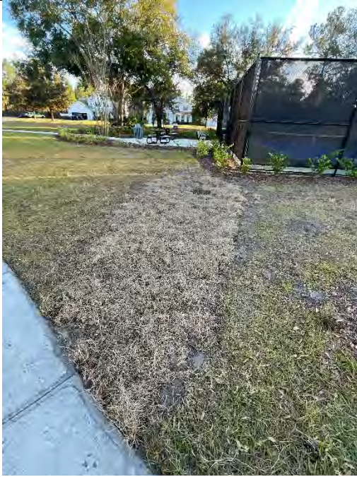
Sitework: Sod Repalced @ Sports Courts
