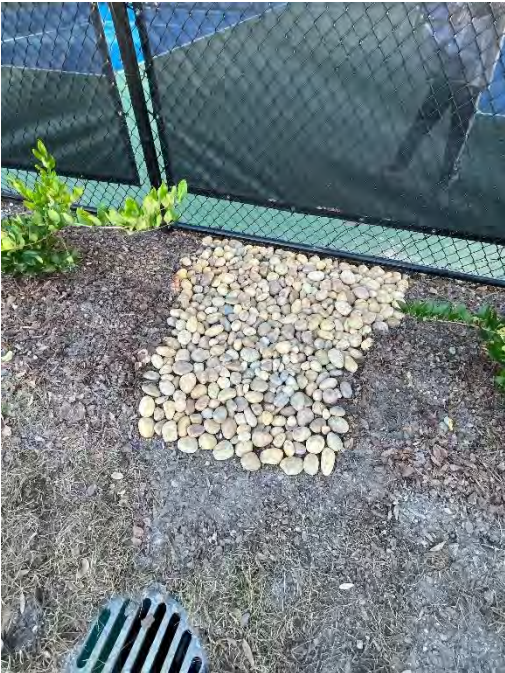
Sitework: Rock Placement @ Sports Courts
