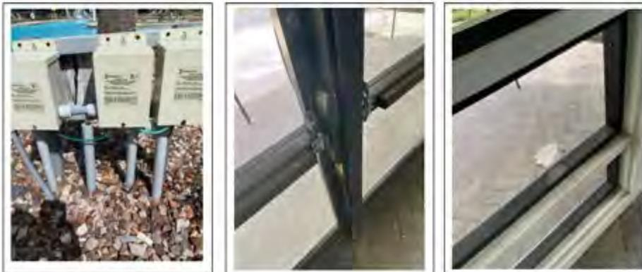
The ground cable on the low-voltage transmitter box on the pool deck is exposed. It should be reinstalled through the conduit for protection, especially in a wet environment. The exposed latches on the indoor screen are also a safety risk. Additionally, I recommend replacing the crash bar due to multiple rips in the screen and using heavier-duty mesh screening for improved durability.
