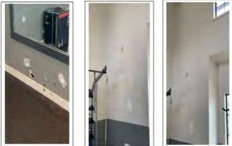
Multiple holes are located throughout the gym. To avoid this issue going forward, I recommend patching holes and installing diamond plating on walls afterward.
